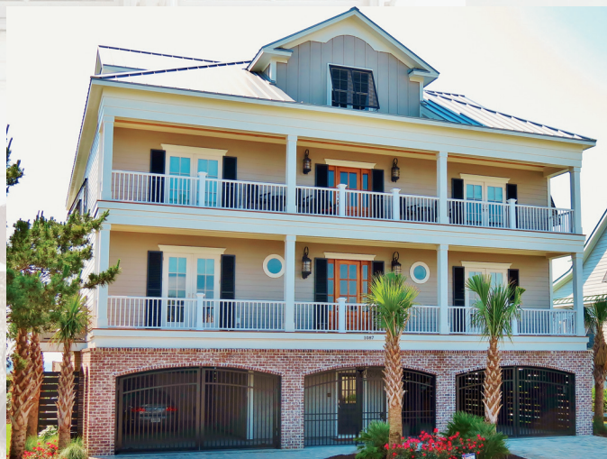
Burroughs Shutter Company installed Colonial Shutters and Bahama Shutters to this Garden City Beach ocean front home.
