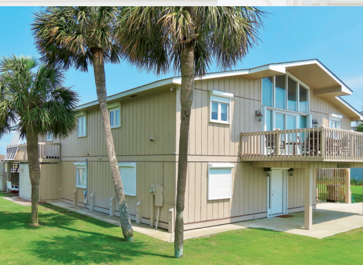
Burroughs Shutter Company installed Roll Down Shutters and Bahama Shutters to this Garden City Beach home.
