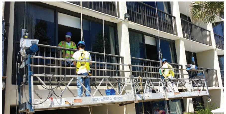
Here the team at CRM is working to remove and replace exterior window glazing at Peppertree Ocean Club in North Myrtle Beach, South Carolina. With expert training in all types of scaffolding CRM is able to reach the exterior of any level for needed repairs and maintenance.
