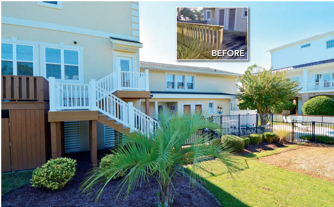
Dynamic Construction, Inc. built the stairwell on the rear of the new addition leading down to the back patio and pool area. The previous wood decking and rails were replaced with a maintenance free decking and railing system.
