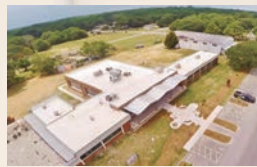
Roofing install for Brunswick Community College completed by Monarch Roofing.
