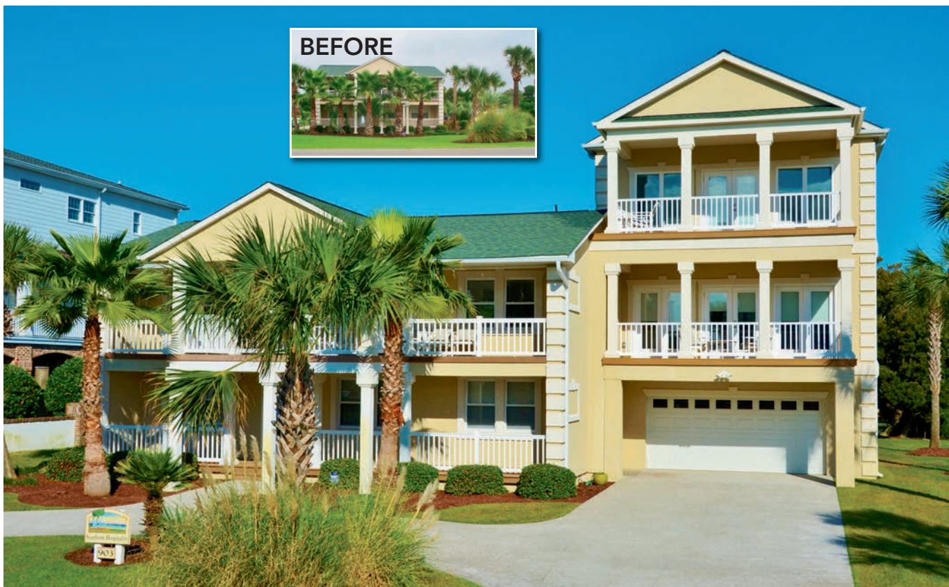
Dynamic Construction, Inc. was responsible for adding on the entire right side of the home including a two car garage. This new addition includes a third story where the master bedroom is now located. Extensive remodeling to the interior of the original home was also completed. The home is owned by Kevin and Kathleen Daly.
