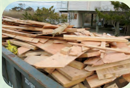
Using extended length wall sheathing reduces the amount of waste at the jobsite. Less waste means fewer trips to the landfill and cost savings.
