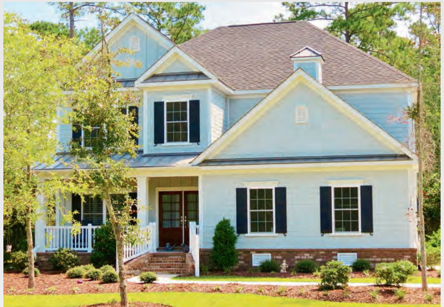
In addition to the James Hardie ColorPlus Lap Siding, Staggered Edge Shake Siding and Board-and-Batten Siding, Contract Exteriors was also responsible for the installation of James Hardie Pediment and Historic Sill around the windows on this Murrells Inlet home.
