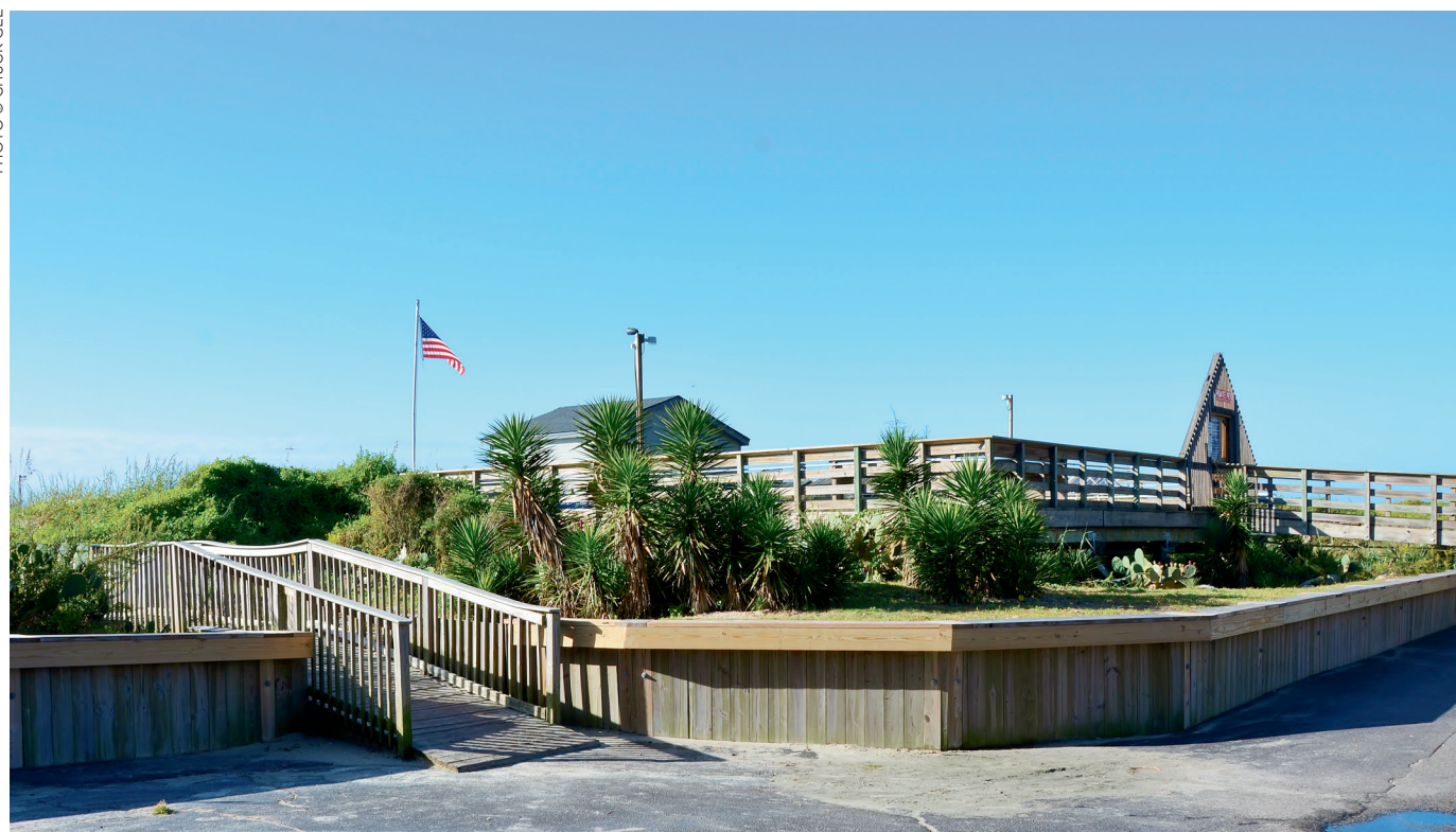
In addition to the pier boards and bench replacements, CCCG also constructed a new pier gate and sea wall-cap.
