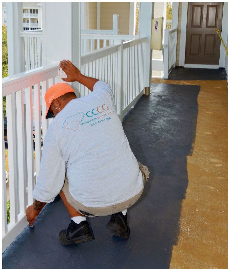
J.P. Pollio (crew leader) applies a water tight membrane to an exterior carpet replacement project in the Carolina Forest area. The membrane installation is applied much like a roof coating in multiple coats and thickens as it dries to provide a rubber like membrane.
