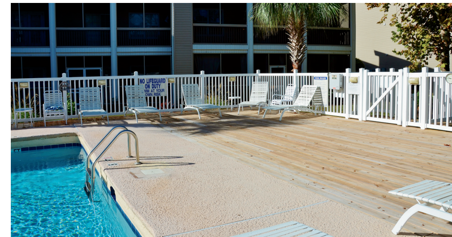
Vinyl fencing's long life span makes it a popular choice for pool areas. CCCG was asked to replace an older wooden fence and decking boards with new vinyl fencing and treated decking boards making this pool area a great place to enjoy the summer in North Myrtle Beach.
