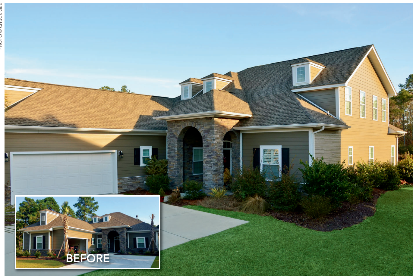
CHC added a raised roof & two additional bedrooms to the residence of Ryan and Katie Neptune. “We tap into the roofline, we match the exact shingle (or other exterior materials), and when we’re done you can’t tell it’s an addition”, says John Melesh.
