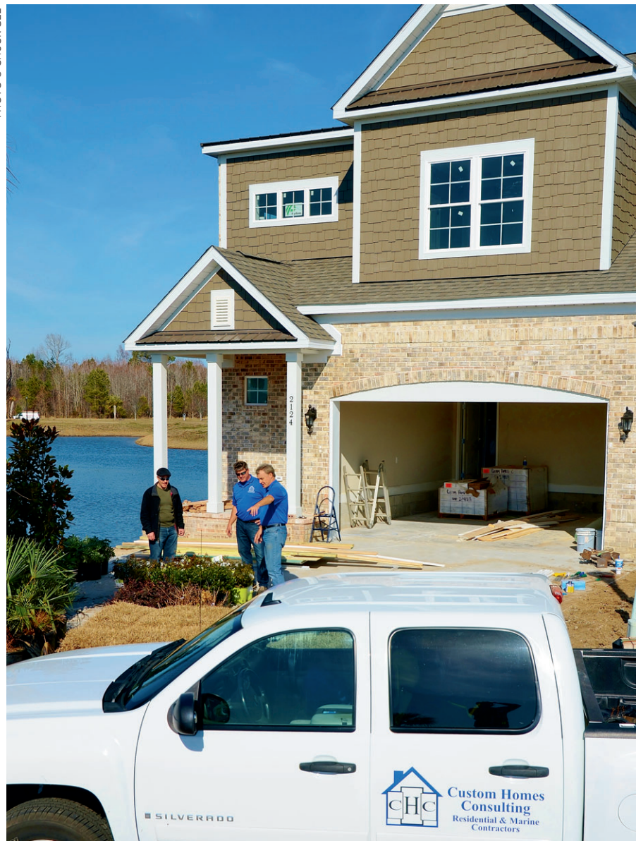
Layne Harris (right) & Steven Quickery (middle) explain the layout of the landscaping package to be completed to new homeowner, Chris Tobin, in front of the home of Chris & Cindy Tobin under construction at Waterway Palms in Myrtle Beach.
