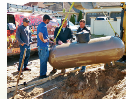
Palmetto Patio & Hearth / Palmetto Propane owners, John Gaddy (2nd from right) & Stevie Bryant (far right) discuss the plans to bury a propane tank for a recent project.
