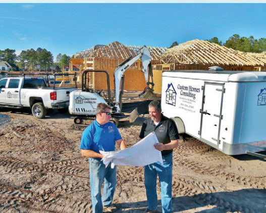
Steven Quickery (left) & Jeff Chestnut (right) on a marine construction jobsite in Plantation Lakes in Myrtle Beach.
