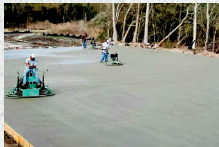
Completing a monolithic slab commercial project.
