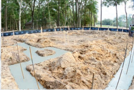
A concrete footing project.
