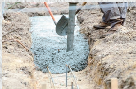
Concrete pumping process.
