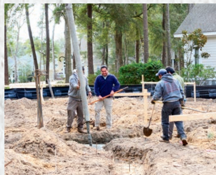
Members of the Professional Concrete, Inc. skilled team prepare concrete footings.
