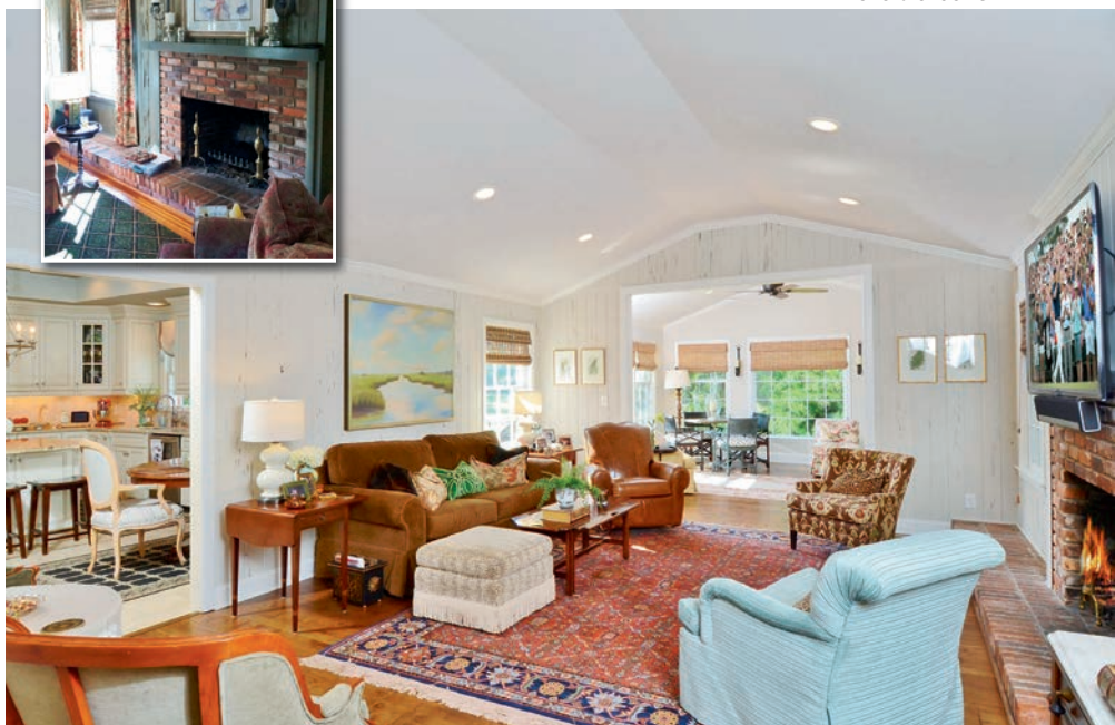
Re-Builders converted the previous 8 ft. ceilings in the Dellinger's den to a 12 ft. vaulted ceiling and installed a 9 ft. tray ceiling in the sunroom. The area was painted and new wood flooring was installed. Re-Builders also repaired and installed pecky cypress walls, new lighting, and relocated the TV area seen above the existing brick fireplace.
