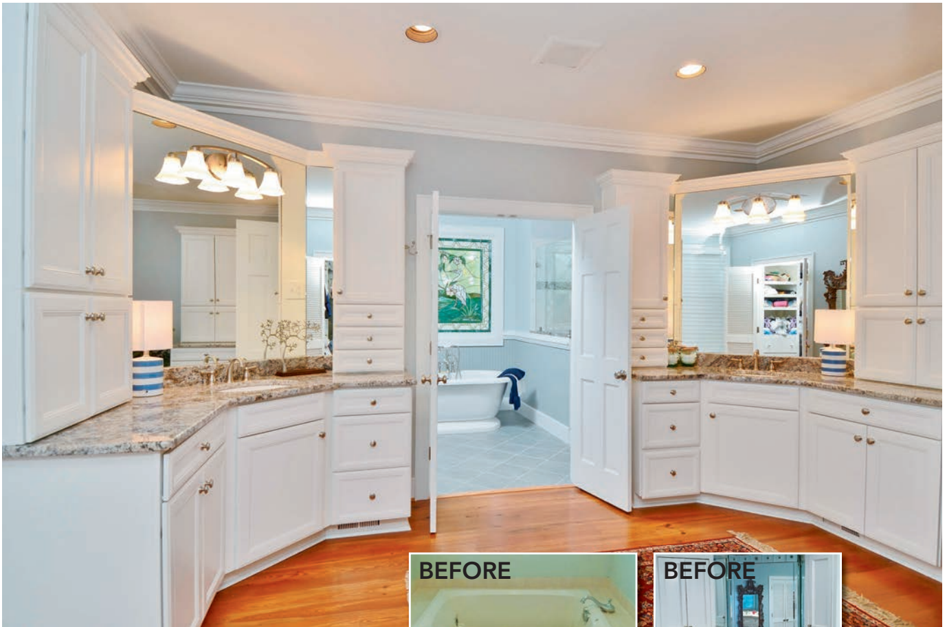
The residence of Oma Hodges. Re-Builders removed the existing whirlpool tub and steam shower along with the vanity cabinets and installed new vanity cabinets with granite counter tops, mirrors, and lighting. A new pedestal tub and new tile shower with bench seat, frameless glass, and recessed soap/shampoo niche was also installed to complete the project.
