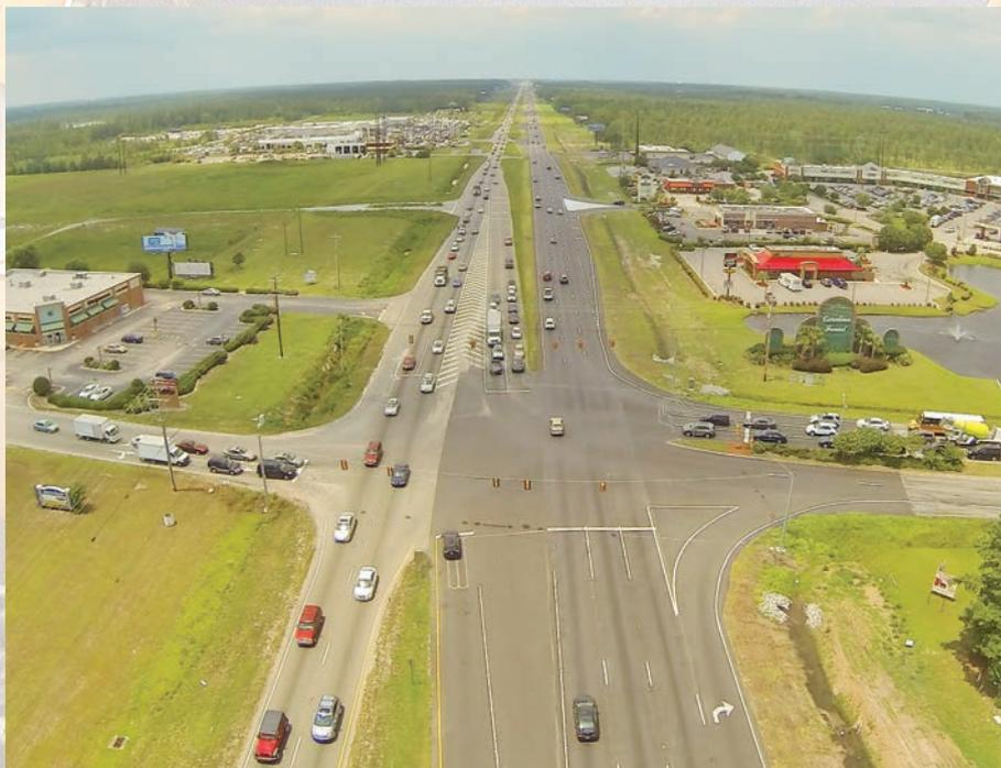
An aerial view of the Highway 501 Widening project Palmetto Corp completed in May 2014. Palmetto Corp crews widened a 2.1 mile stretch of the northbound lanes from two lanes to three.
