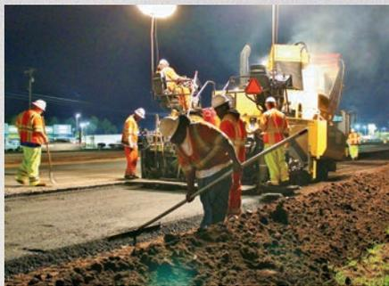
A Palmetto Corp crew paving the new third lane on Highway 501. Because Highway 501 is a highly trafficked roadway, all work had to be performed at night.
