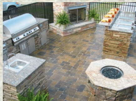
Ford's Fuel & Propane specializes in designing and installing outdoor kitchens.
