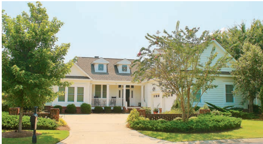
This lovely Cottage at the Reserve sits in a well-manicured lowcountry community and is a testament to the timeliness of a home...or cottage...built by Classic. Attention to detail, both inside and out, along with superb craftsmanship, makes this a home that will be in the family for generations. Classic is currently finalizing plans for another home in The Cottages at the Reserve .
