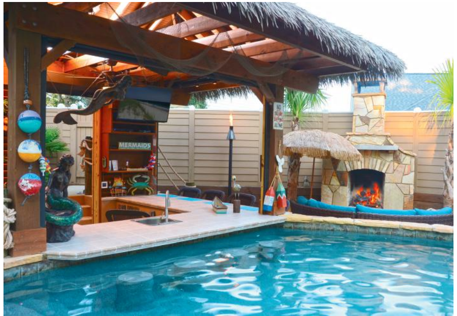
Calibre Development was responsible for the installation of this sunken outdoor kitchen & living area. This project included installing a tiki hut, walkways, bollards & rope handrails. A critical part of this process was determining the correct drainage and precise elevations.
