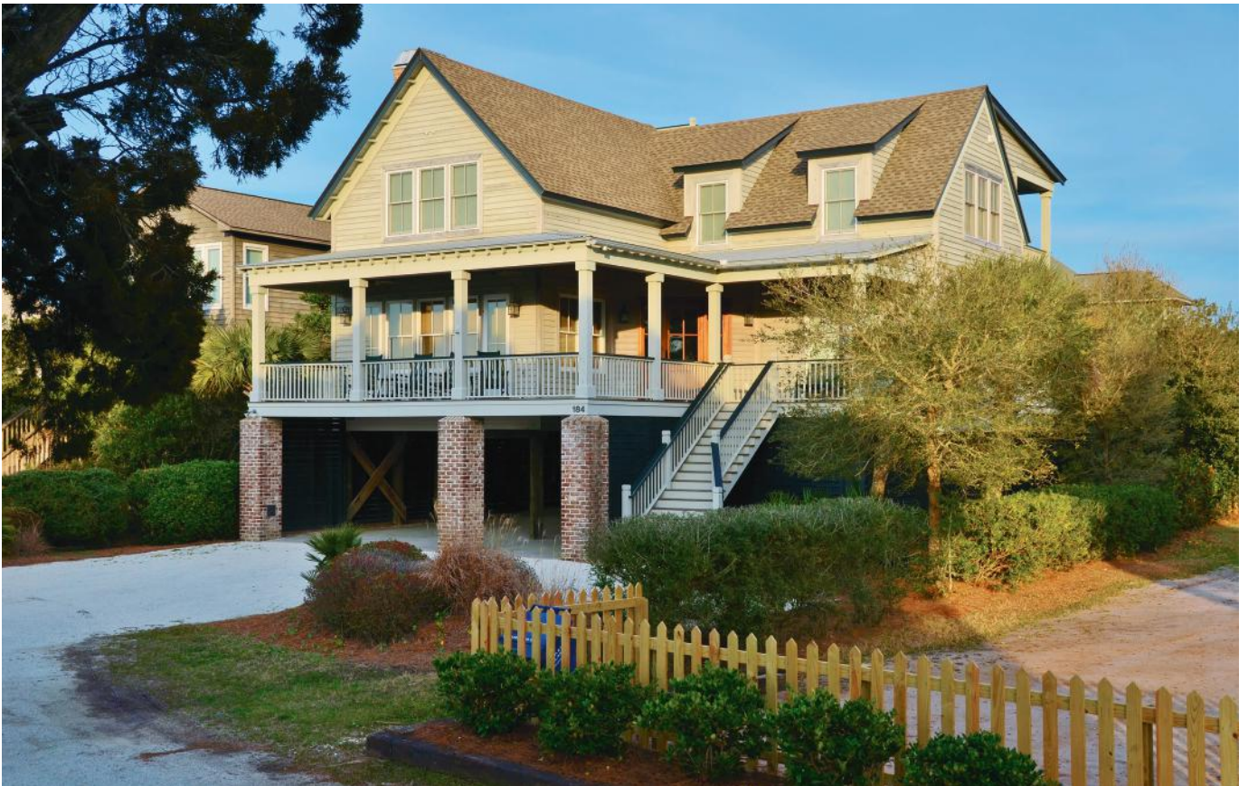
The view from the marsh in Pawleys Island of a custom home built by Calibre Development. Calibre installed beautiful cypress siding on the exterior of this home.
