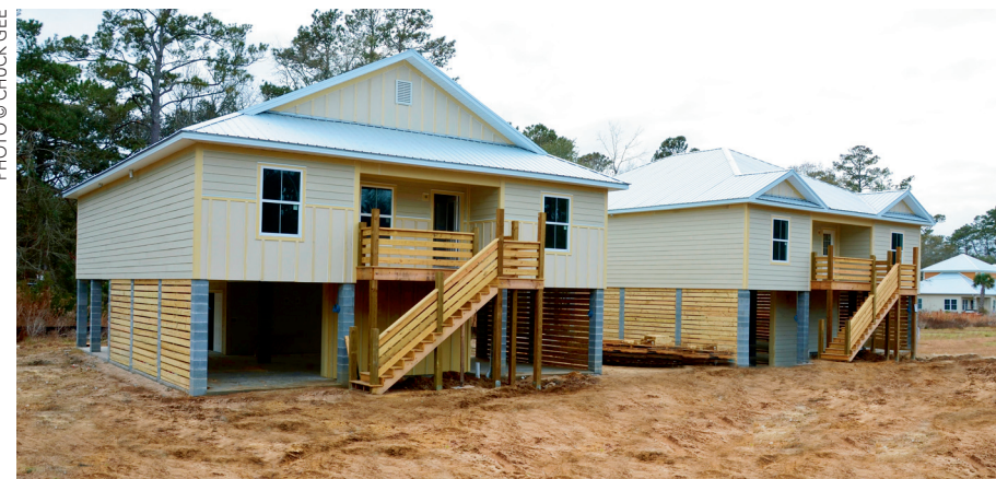
The new Pawleys Sunset community under construction.
