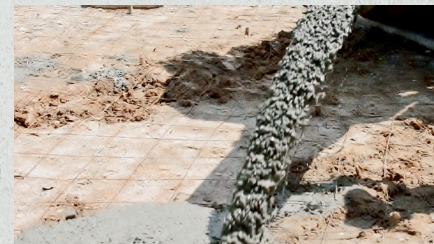
Thomas Concrete is currently introducing their new 'Carbon Cure' technology.
