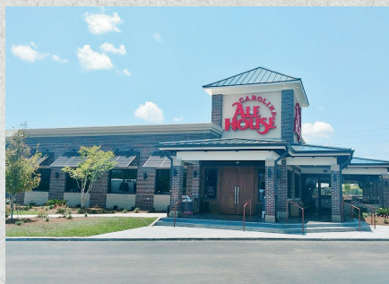
East Coast Masonry & Stone handles a lot of commercial construction.
