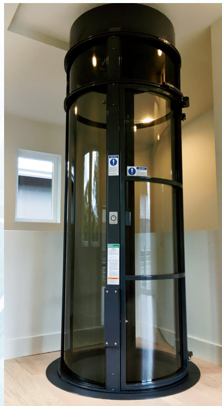
The Pneumatic Vacuum Elevator (PVE) has become increasingly popular to install in existing homes that were not originally built to accommodate a traditional elevator shaft.
