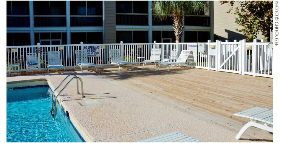
Vinyl fencing's long life span makes it a popular choice for pool areas. CCCG was asked to replace an older wooden fence and decking boards with new vinyl fencing and treated decking boards making this pool area a great place to enjoy the summer in North Myrtle Beach.
