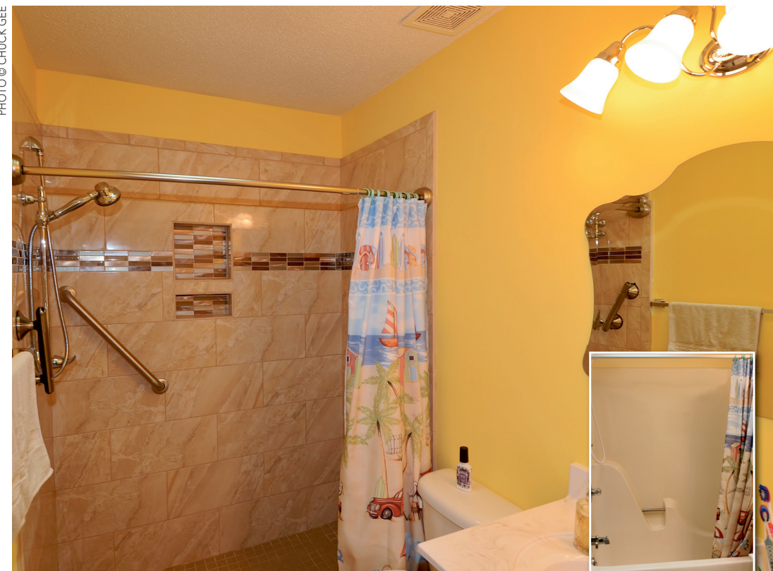
The guest bathroom at the Passarella residence was completed in early September of 2017, which included new vanity cabinetry, and a ceramic tile shower.
