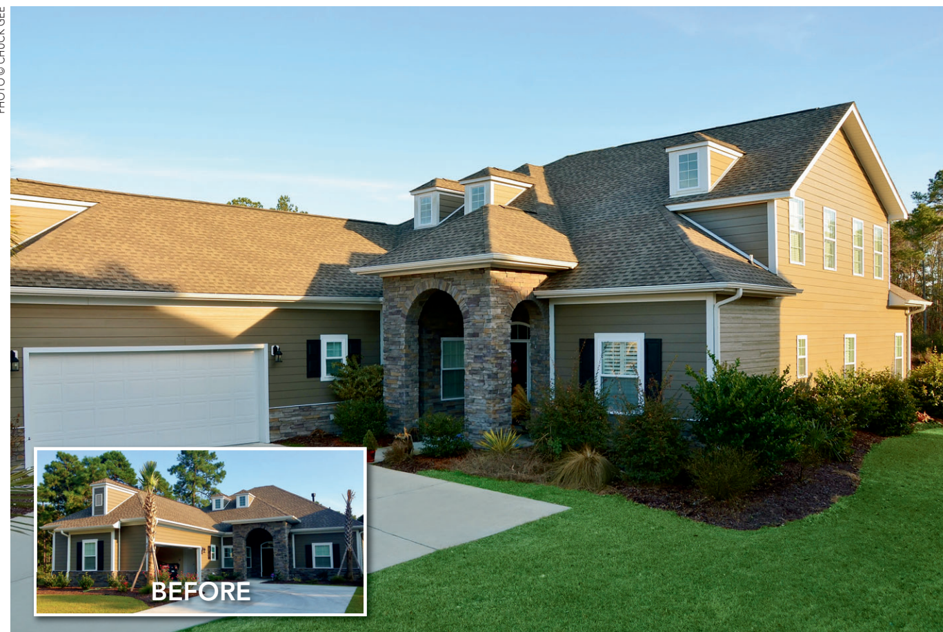
CHC added a raised roof & two additional bedrooms to the residence of Ryan and Katie Neptune. “We tap into the roofline, we match the exact shingle (or other exterior materials), and when we’re done you can’t tell it’s an addition”, says John Melesh.
