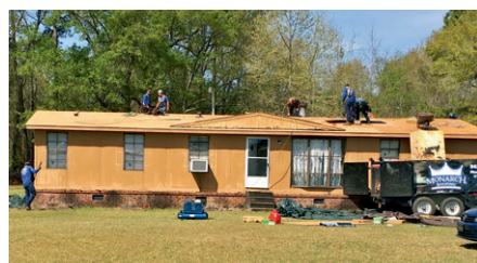
The Monarch Roofing team removed Miss Shirley Hughes' old roof & installed a brand new roof on April 6th.
