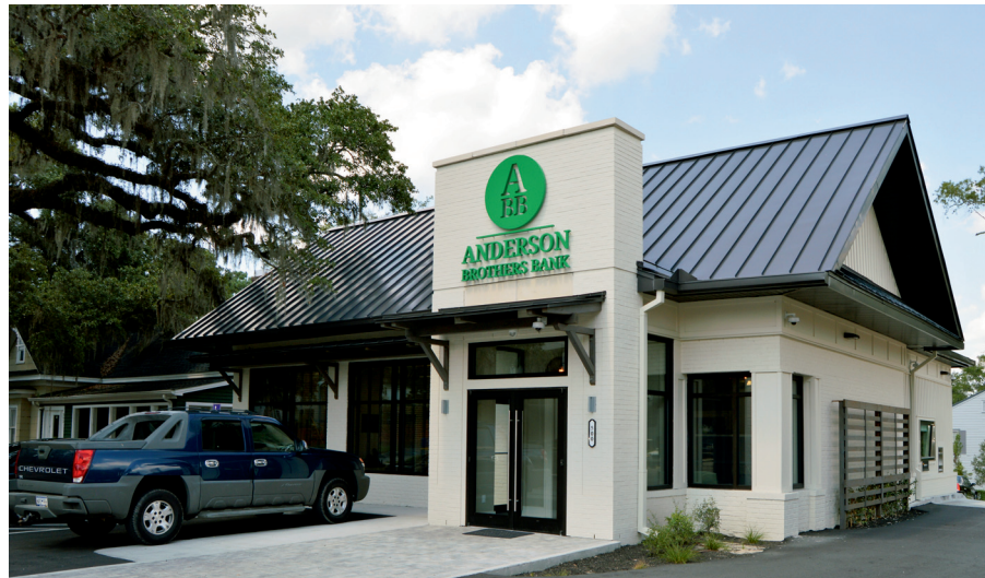
Tungsten was responsible for the demolition of the previous building @ this property located on Main St. in Conway in order to build the new Anderson Brothers bank. This project included a new retaining wall to accommodate the parking, a renovation including a simple gable roof with feature entries on both the front and back of the building. The bank was competed with metal roofing, painted brick, custom brackets, awning supports and a green wall, as well as custom millwork on the inside. This building ended up winning an award from Conway Downtown Alive.
