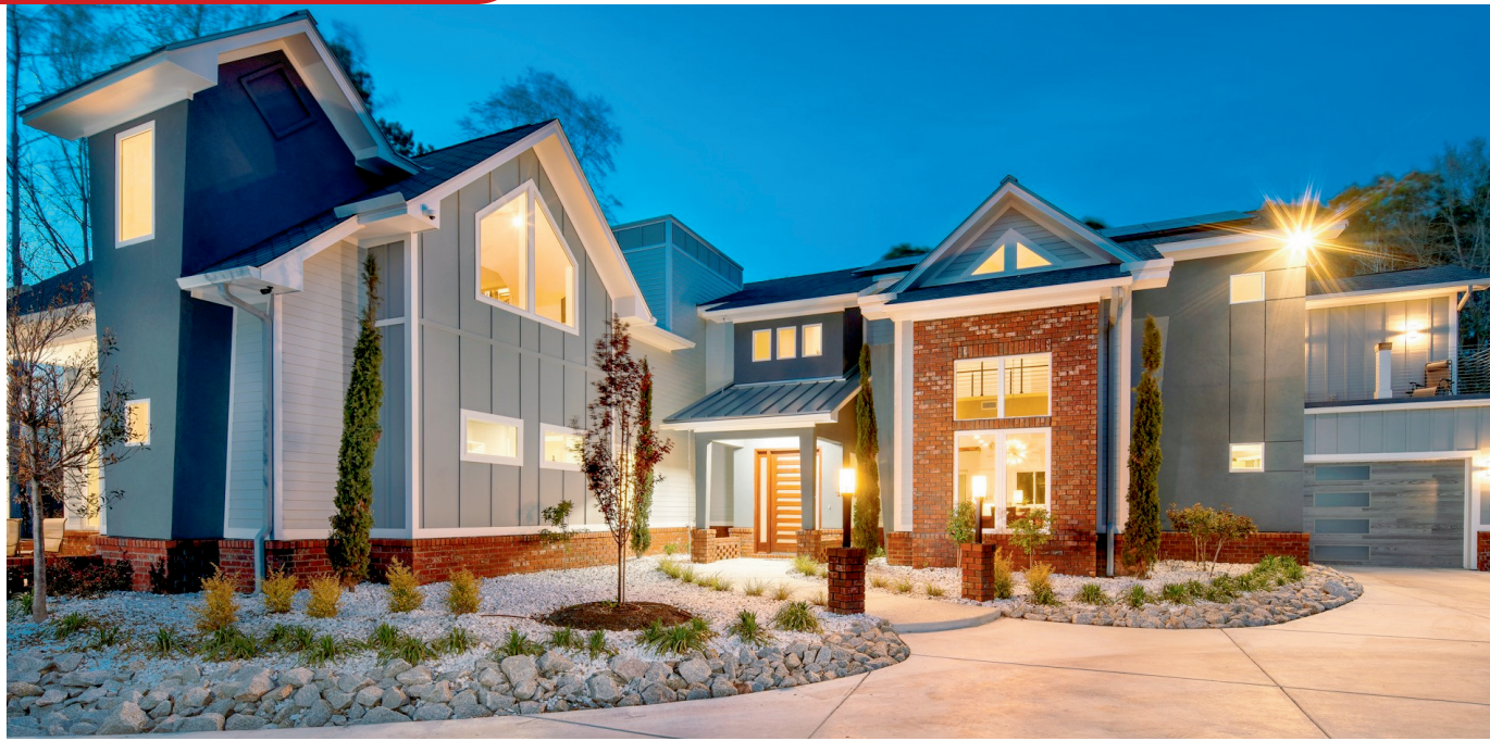
Tungsten utilized a nice balance between clean modern lines and traditional materials on this residential home. The exterior finishes included sand faced brick, EIFS, Hardie siding, Hardie board and batten, as well as a mix of shingle roofing with metal accents and a custom front entry door.
