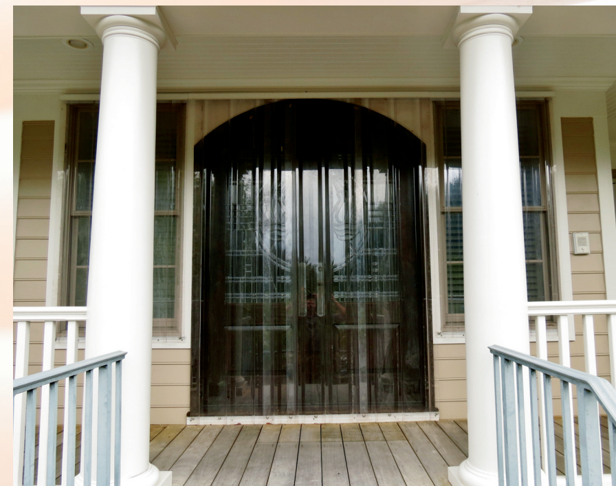
Clear Storm Panels cover the front door of this beach home in Pawleys Island, SC.
