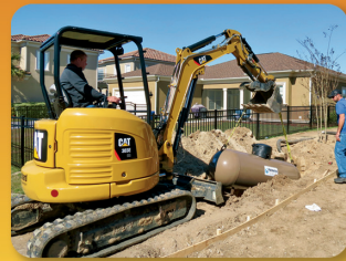
New Construction Natural Gas & Propane Lines
