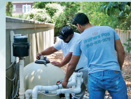
Brothers Pool Construction also handles the design & installation of the pump configuration for pools if needed.
