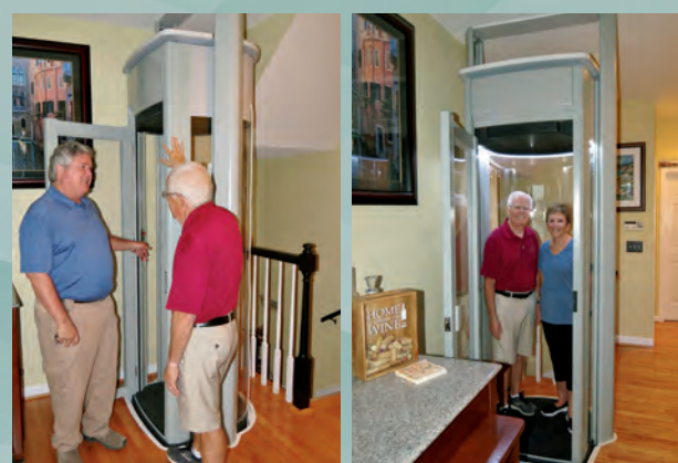
Stan Godshall (left) reviews the ease of operation for the Stiltz Lift with homeowner, Bill White. Bill and his wife Pat are very pleased with their experience with Port City Elevator and their decision to have the Stiltz Lift installed in their existing home in Tidewater Plantation. The existing structure could not accommodate a traditional elevator shaft, so the Stiltz Lift was a welcomed option to meet their needs.
