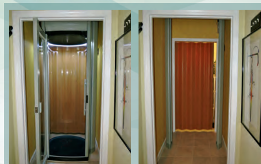
Homeowner's Bill and Pat White are still able to access their closet downstairs when the Stiltz Lift is moved to the 2nd floor.
