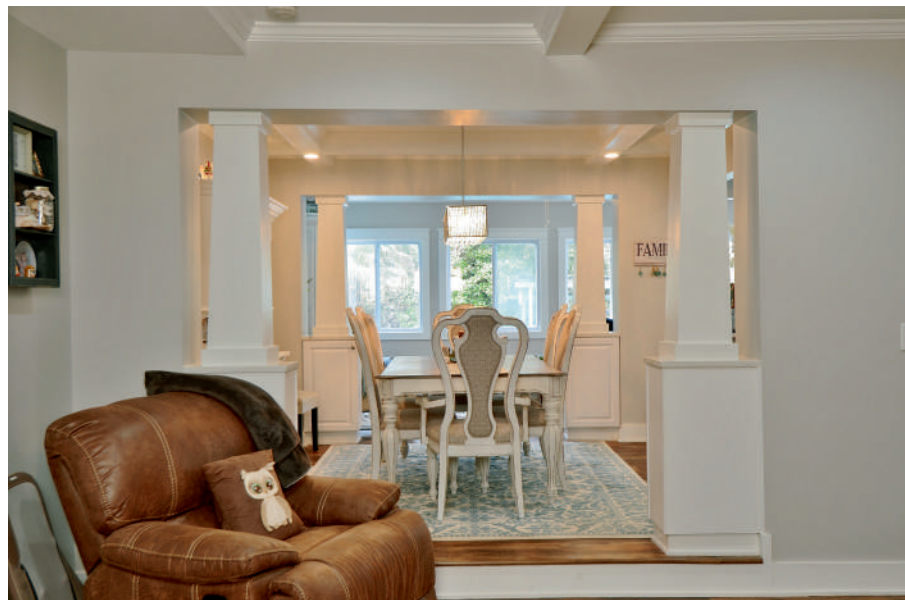
Jon Harrah was responsible for adding a coffered ceiling with red lights, and Craftsman columns with cabinet storage in the Ritchie dining room area.
