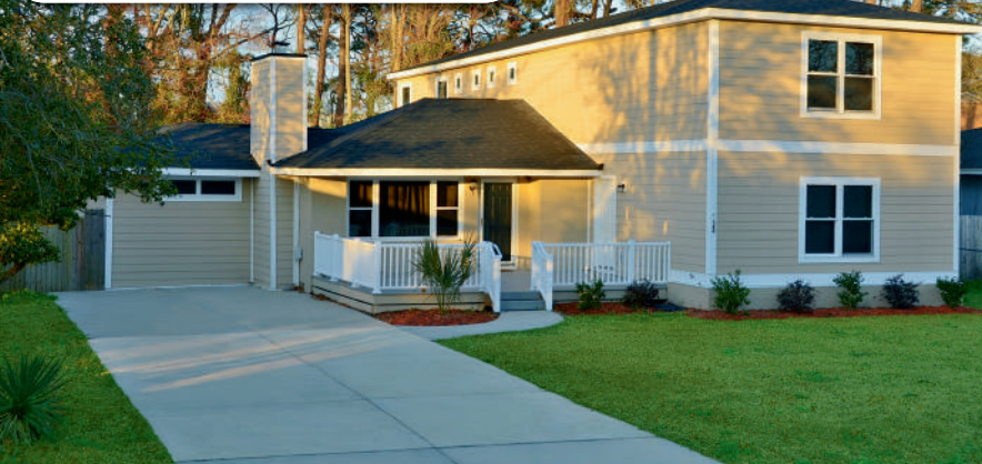
Jon Harrah was responsible for adding 2000 square foot of living space to this existing 1300 square foot home in Myrtle Beach, SC. Because of space limitations, the new addition had to be added to the top of the existing structure in order to expand the square footage. This home was originally built in the 1950’s. Homeowner, Ramon Arbaiza, was very comfortable in knowing that Jon “knew all of the rules and regulations from working with the city”. Once the job started, it was completed in less than four months.
