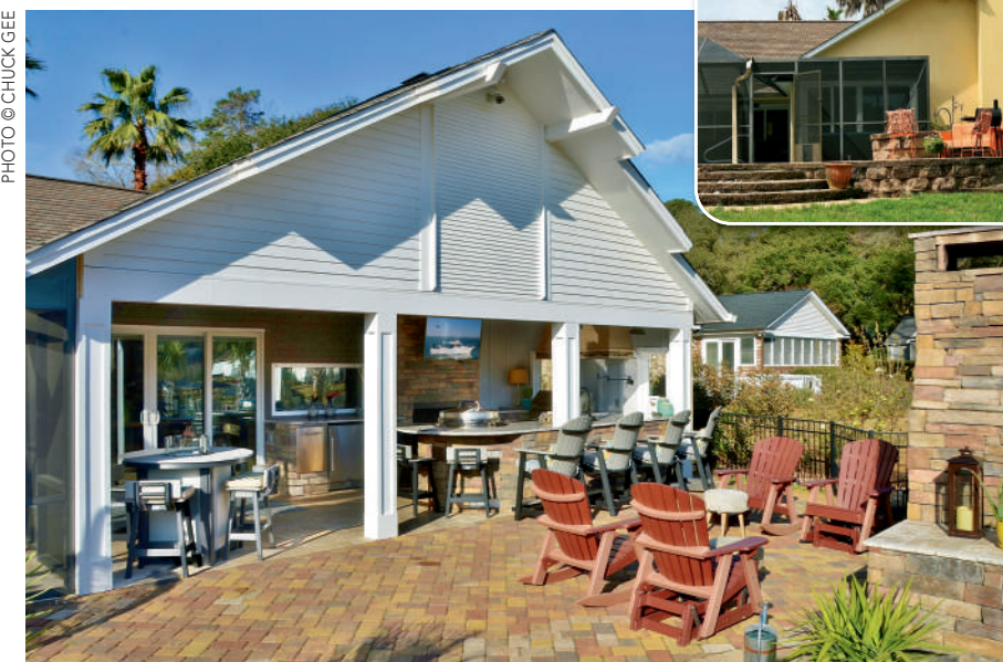
Jon Harrah was responsible for completing the total remodel/renovation of the rear of Lisa Phillip’s home in Mt. Gilead. An exterior wall needed to be added on one side (with matching stucco) so the roof could be extended over the space (with matching shingles). The design included a hibachi grill, sink, two refrigerators, lighting, and an overhead fan. Travertine was used on the floor. “Jon is a great contractor and I would highly recommend him. He did a beautiful job and fulfilled everything that was requested in a timely manner”, said Lisa.
