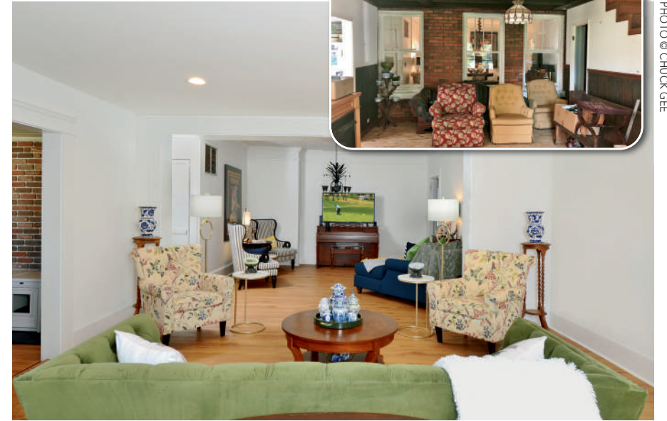
Jon Harrah was responsible for the removal of the existing original 1950’s double wythe brick wall and windows to extend the living area. The stairs to the 2nd floor (seen in the BEFORE Photo to the top right) were relocated to the exterior of this home, in Loris, SC, to create more living space. Homeowner, Maria Worley was very pleased with the completed job. “I did not even think about creating one big room. I wanted to carry over the brick into the kitchen to kind of blend it. Jon asked if I’d ever thought about removing the brick wall and enlarging the space”, said Maria.
