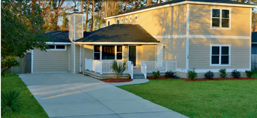
Jon Harrah was responsible for adding 2000 square foot of living space to this existing 1300 square foot home in Myrtle Beach, SC. Because of space limitations, the new addition had to be added to the top of the existing structure in order to expand the square footage. This home was originally built in the 1950’s. Homeowner, Ramon Arbaiza, was very comfortable in knowing that Jon “knew all of the rules and regulations from working with the city”. Once the job started, it was completed in less than four months.
