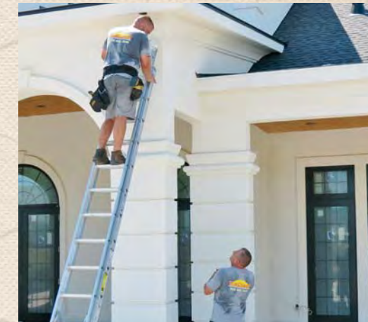
Darryl Hill (standing in photo) and his son Zeb Hill (on ladder) have become two highly respected gutter installers across Horry & Georgetown Counties.
