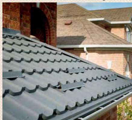
Worthouse metal roofing
