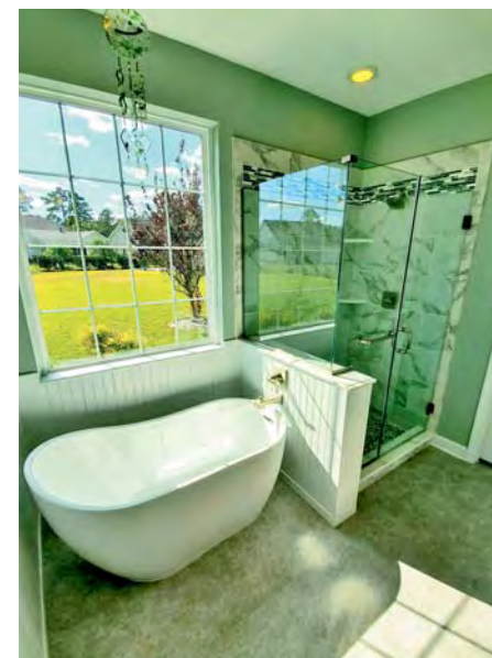
Conway Builders remodeled the master bathroom in the Remmert residence. They removed the existing built in soaker tub & shower stall, & installed a new tile shower with frame-less glass surround & a linear glass accent. To complement the new shower, they installed a free-standing soaking tub and new EVP flooring. The shower now has a quartz corner seat and curb to match the new selected tiles & Delta fixtures in brushed nickel.
