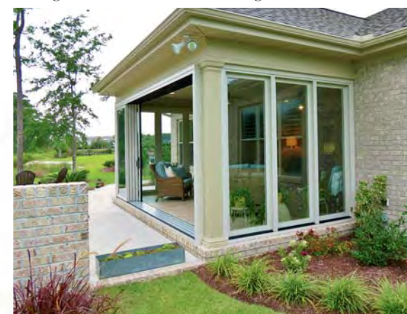
Cove Construction was responsible for installing these Fixed Panel Doors to the right & left of this sunroom, which are a part of the Pella® Architect Series.
