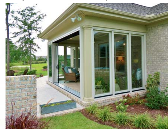
Cove Construction was responsible for installing these Fixed Panel Doors to the right & left of this sunroom, which are a part of the Pella® Architect Series.
