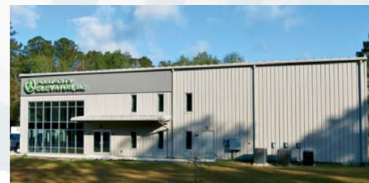
The Port City Elevator's corporate office located @ 5704 Nixon Ln. in Castle Hayne, NC. Port City Elevator services the Horry & Georgetown, SC markets.
