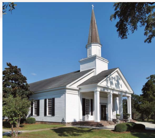
Burroughs Shutter Company installed Colonial shutters on Belin Memorial United Methodist Church in Murrells Inlet, SC.
