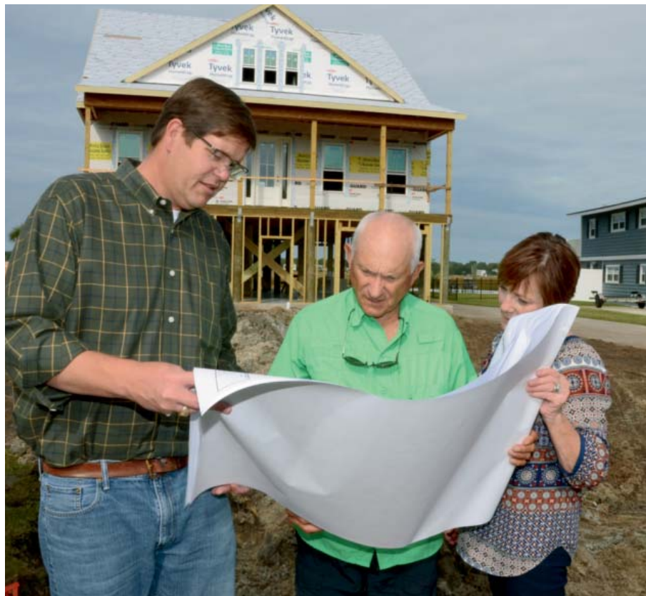
Drew Hanna (left) reviews the plans with homeowner's Woody & Nancy McKay in front of their home under construction in Garden City, SC. "We're pretty much building the same five bedroom house we had at Collins Creek Landing. We loved the layout and asked Drew if he could do it on 15' pilings." While still living at Collins Creek Landing Woody and Nancy watched 8 or 10 houses being built by Port City Homes and were impressed with their process. Woody said, "It was one crew after another. There was never any downtime. I thought, 'that's the kind of guy I want to build my house.'" Woody said, "We're just crazy about Drew and his family."
