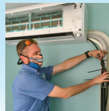
The installation of the interior high efficiency mini split system equipment
