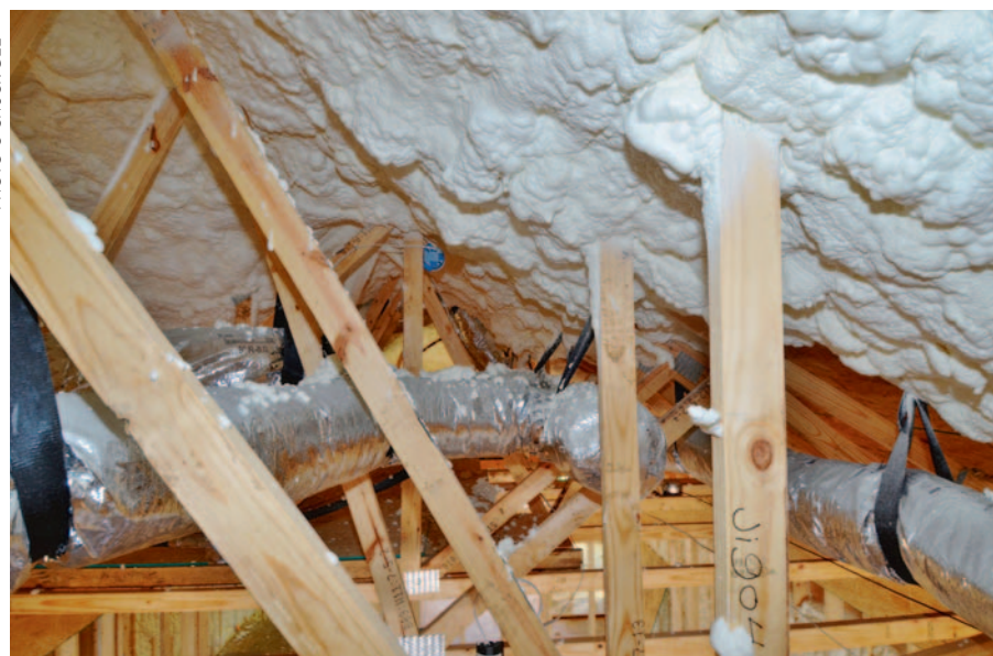
As a result of the surrounding spray foam insulation, the HVAC components in this attic are now in a conditioned space.
