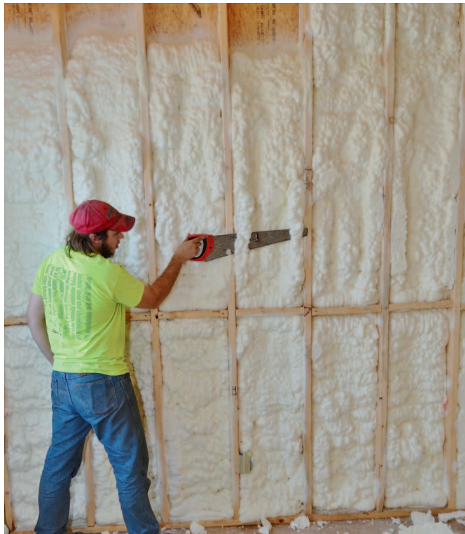
The clean up process after the spray foam insulation is applied.
