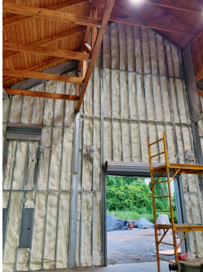
Spray foam insulation can be applied to metal buildings as well as traditional stick built buildings and is equally effective for both types of construction.
