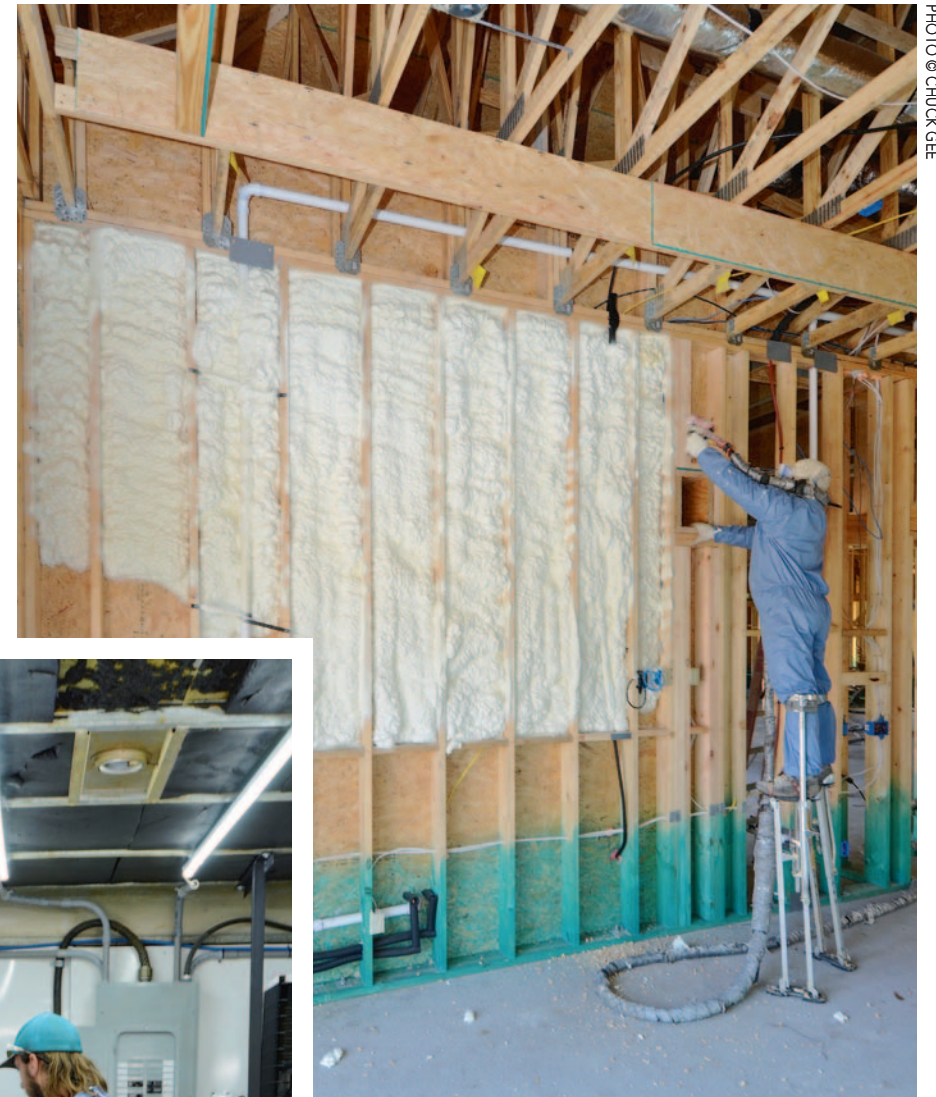
The application of 'Open Cell' spray foam insulation at a custom home in Cypress River Plantation. “'Open Cell' spray foam insulation is the most economical and has a lesser R-value per inch,” says Relford.
