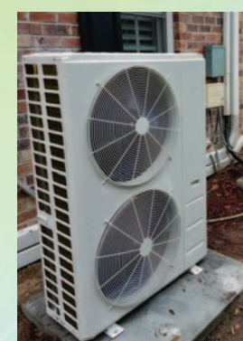
The exterior of a high efficiency mini split system
