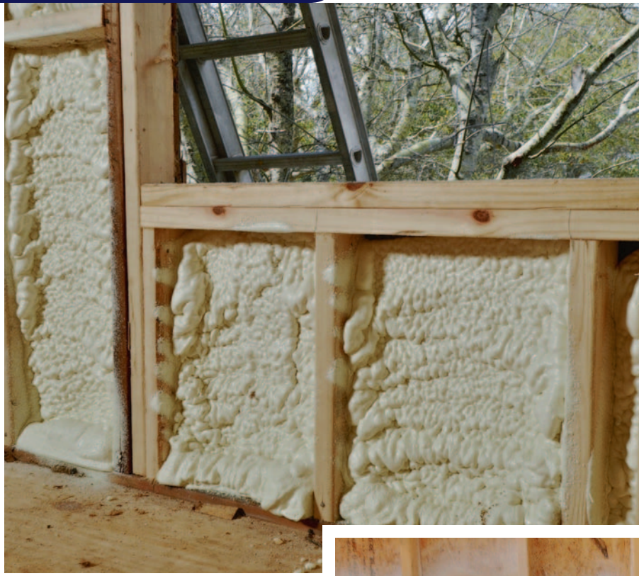
The application of 'Closed Cell' spray foam insulation before the completion of the interior walls in the construction process.
