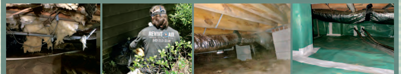
Revive Air was hired to remove all of the existing insulation & seal the crawl space under this residential home in Myrtle Beach.
