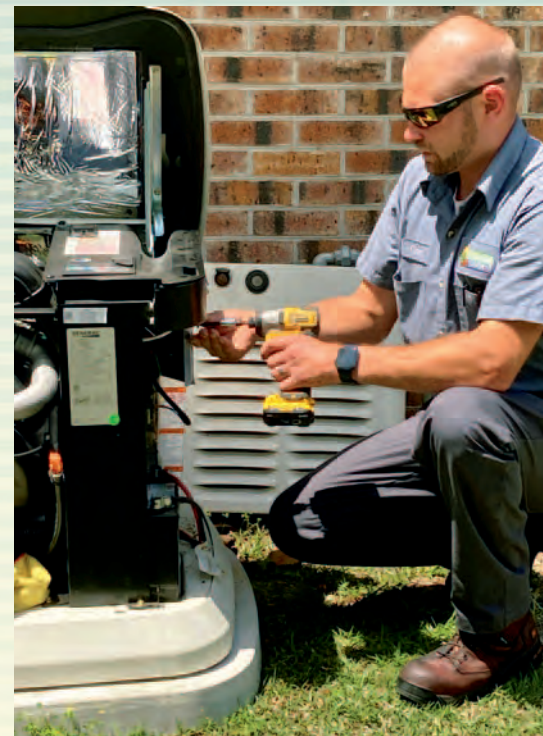
A Carolina Cool service technician performs maintenance on a residential standby generator.
