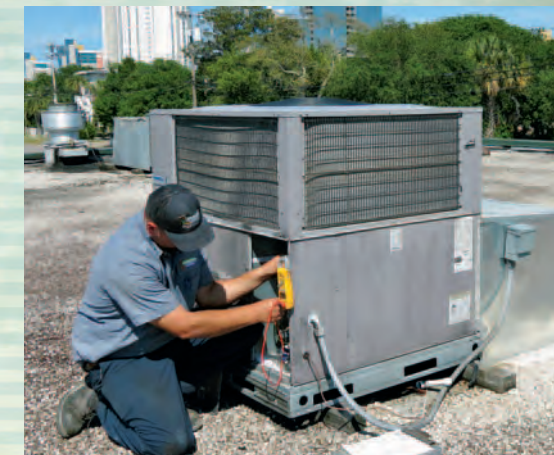
A Carolina Cool service technician performs maintenance on a rooftop unit @ a Myrtle Beach restaurant.
