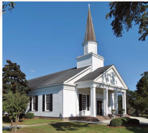
Burroughs Shutter Company installed Colonial shutters on Belin Memorial United Methodist Church in Murrells Inlet, SC.
