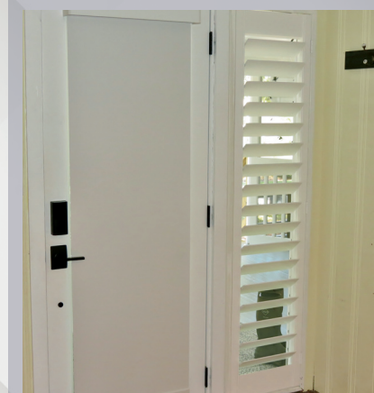
Interior solar shades can be utilized on windows as well as doors.
