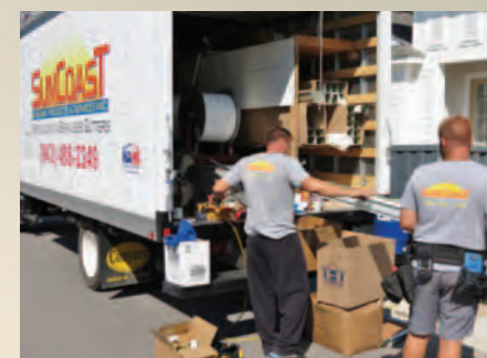
Darryl Hill (left) & Zeb Hill (right) measure and cut the custom gutters for a project in Ocean Isle Beach, NC.
