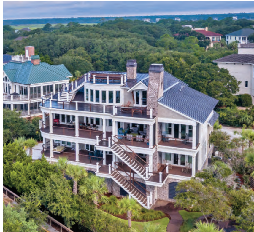
The rear of the residence of Jim & Peggy Morgan in DeBordieu Colony. This home was designed by Catalyst Architects. "I'll be honest with you...I can't say enough about Robert, his father, Bob, and their subcontractors and crew members. They almost became my family. And we learned very quickly that they stayed with the house. If a question comes up, it doesn't matter whether it's a month later or two years later, they want to hear about it and will do something about it," says Jim.
