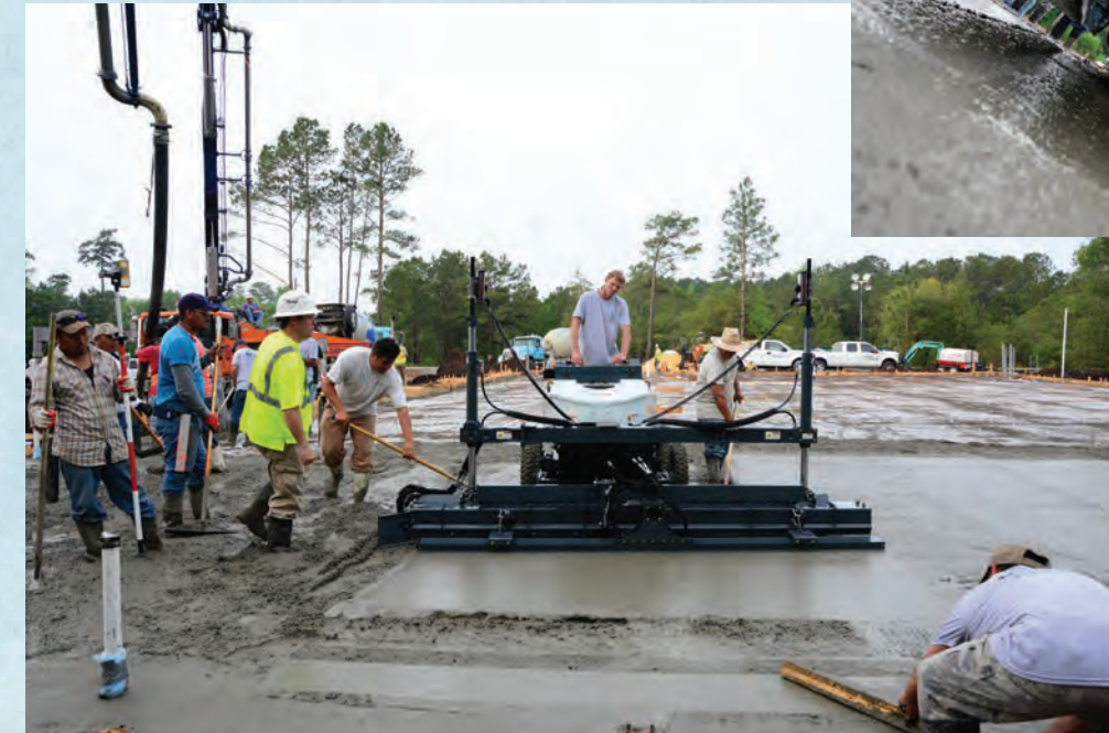
Professional Concrete's 3-D Laser Screed Machine
