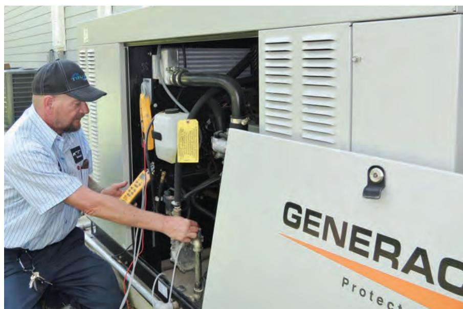
Generators are extremely popular in this coastal market & Trusted Home Services installs & provides maintenance for them throughout the area.
