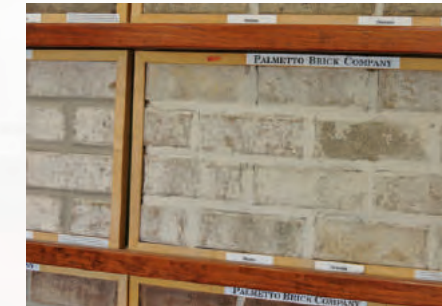
According to Redwine, the flushed old world brushed mortar joints have become popular as of late.
