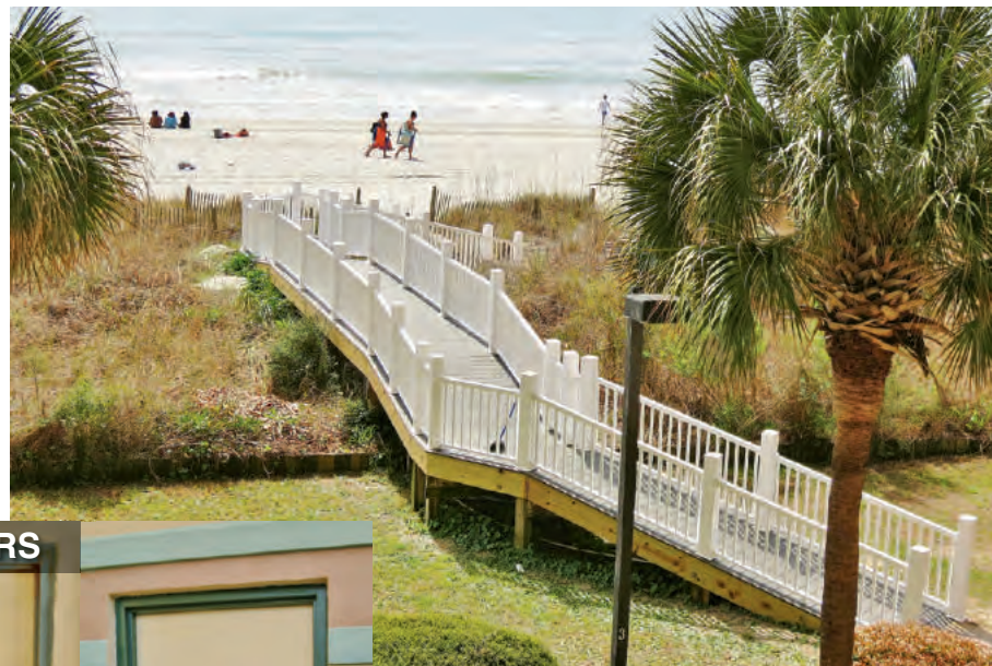
Allstar Construction Services completed the renovation for this walkway in North Myrtle Beach for the management company that handles this high rise vacation rental complex. They replaced the old treated wood with composite Trex decking, PVC posts & pickets.
