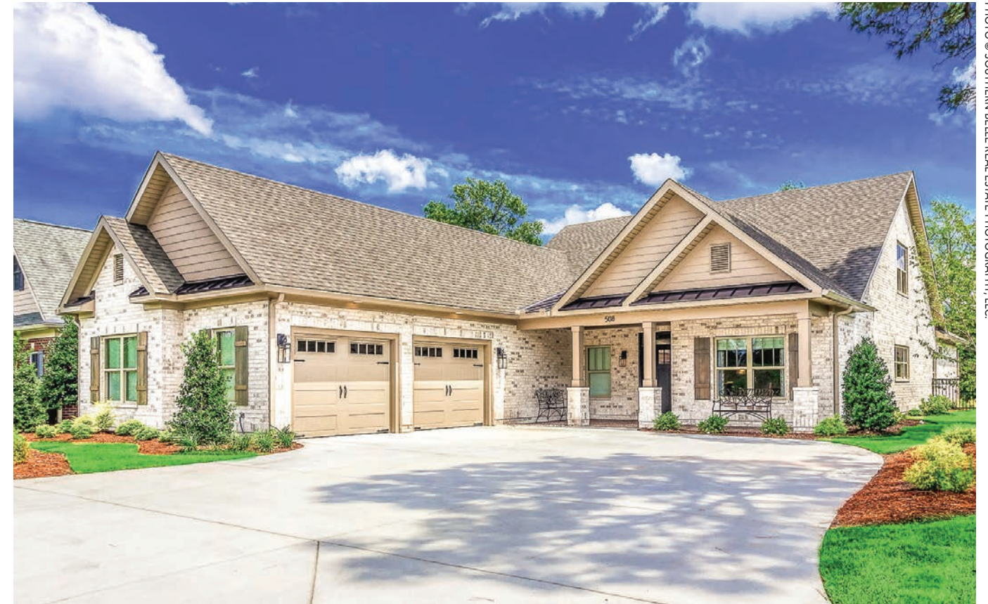
The Quirk residence features Riviera brick exterior and sleek standing seam metal roof accents. The striking combination of textures and colors creates a unique and sophisticated look that is both timeless and contemporary.
