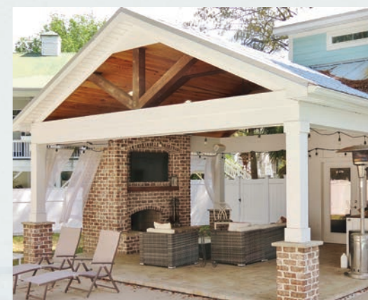
Palmetto Brick furnished the brick for this outdoor living area & Artwork Masonry & Construction was responsible for the installation.
