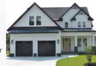
Suncoast Building Products & Services installed the gutters on this home built by MJM Custom Home Building.
