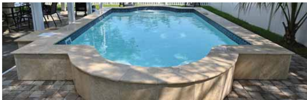
Elko designed this pool partially out of the ground. This helps with water flooding in the yard and also provides additional seating for the swimmers.
