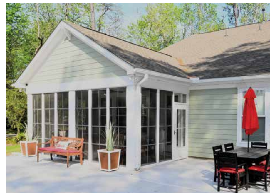
Carolina Bays designs their porch enclosures to allow as much visibility and air flow to the outside as possible. This is the exterior photo of the enclosure shown above.
