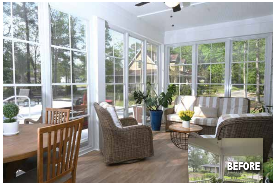
Screen porches are nice, but not usable for large parts of the year due to pollen, rain and cold air. This enclosure, completed by Carolina Bays in Paveleys Island, allowed the customer to have the screen porch, but with all the benefits of an enclosed room.
