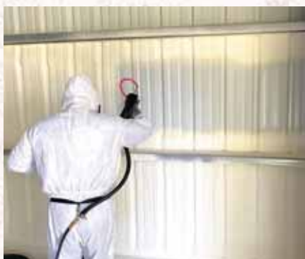
Spray Polyurethane Foam is often used in metal buildings.
